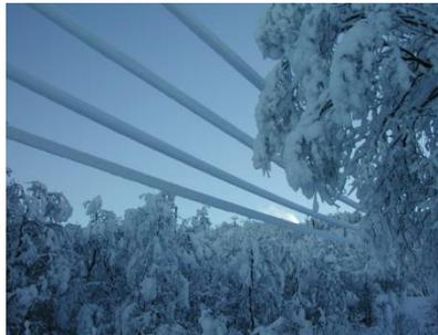
Figure 2: Snow load on power line. Photo Hallingdal Kraftnett
