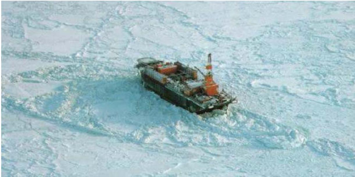
**Figure 4** Photograph of the SSDC at the Phoenix site. Note the large rubble field surrounding the structure (*Timco and Johnston, 2002*)
