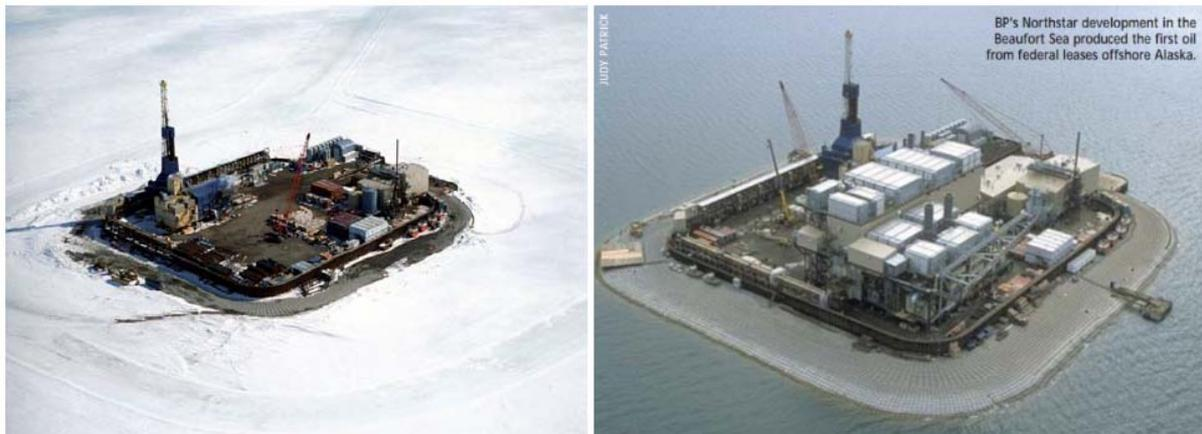
**Figure 16** Northstar production facility in shallow water (photo left: island under construction in winter ice conditions) [source: <http://www.bp.com>]
