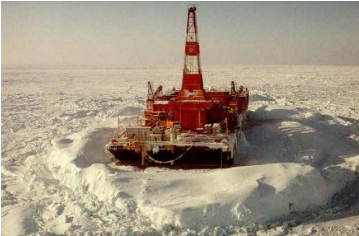
**Figure 3** SSDC at the Kogyuk site in the Beaufort Sea. Sprayed ice rubble is surrounding the structure (*Timco & Johnston, 2002*)
