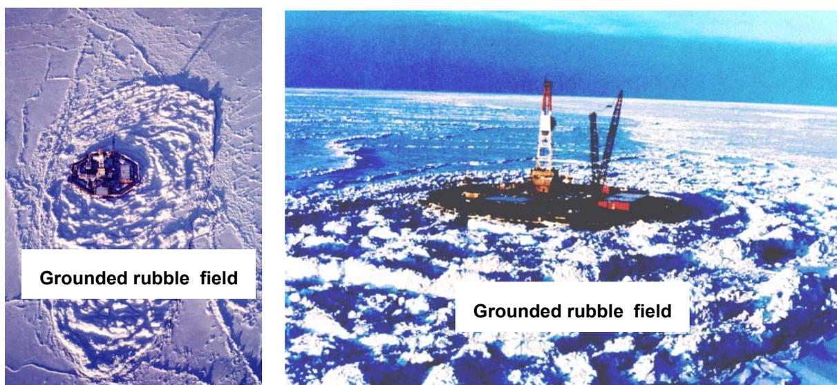
**Figure 6** Grounded rubble field around the CRI at the Kaubvik site (left) and ice rubble surrounding the CRI at the Amerk site (right), [after *Timco and Johnston, 2002*]
