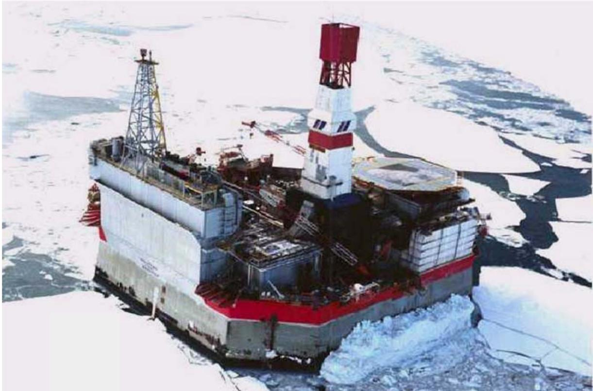
**Figure 7**      **Photograph of the Molikpaq with accumulated crushed ice on upstream side**
