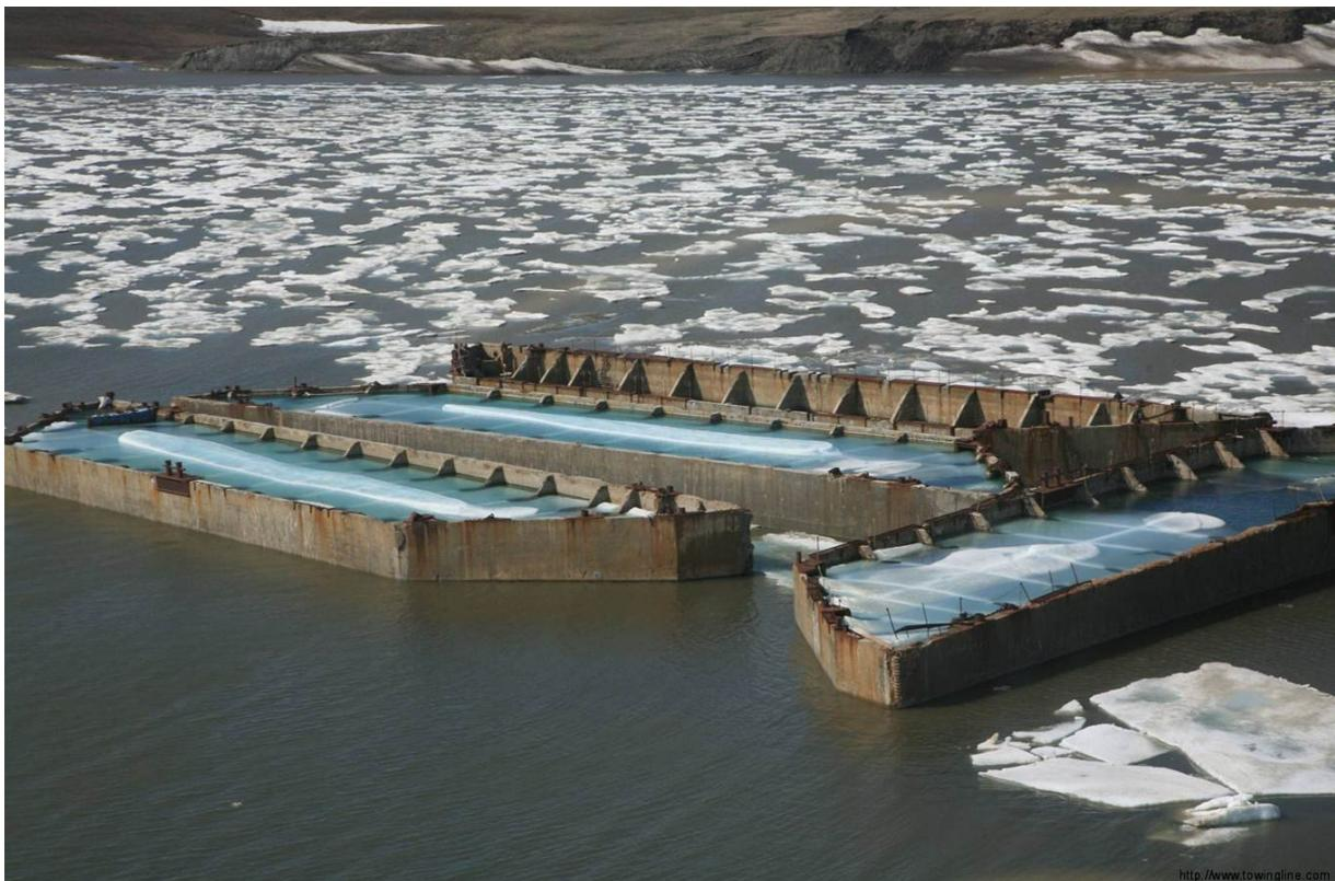
**Figure 9** Caissons floated to the berm of Tarsiut Island
