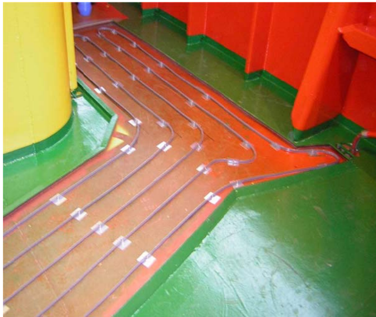
Figure 41 Heating coils to prevent ice accumulation ( Koren, 2007 )
