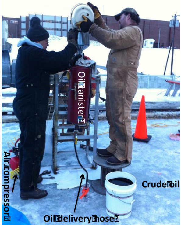
Figure 13. Photograph showing the filling of the pressurised oil delivery system. This system allowed oil to be deployed efficiently and effectively as well as constraining the oil to the experimental hollow under the sea ice. No evidence of oil spreading beyond the hollow was seen.
