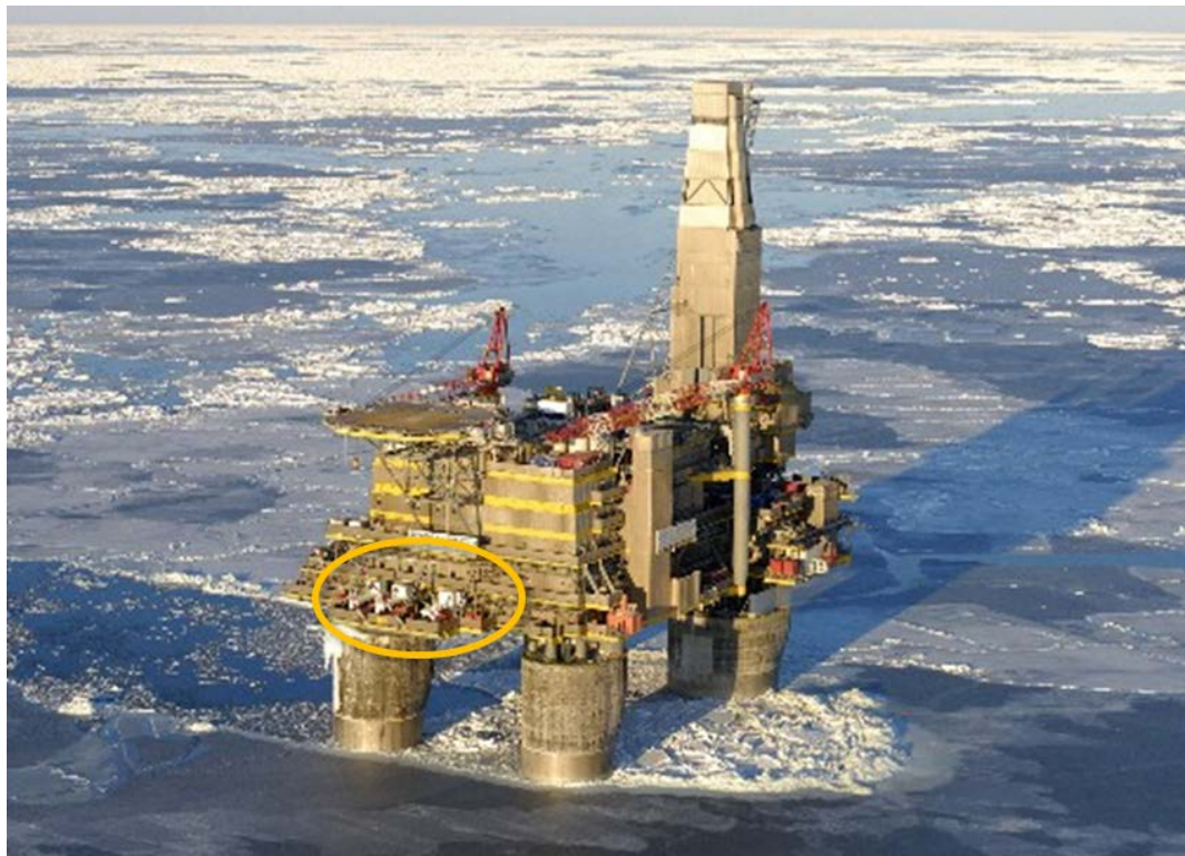
Figure 8-2: Concrete drilling and production platform Lunskeye A in drifting ice (note the marked free fall rescue boats)
