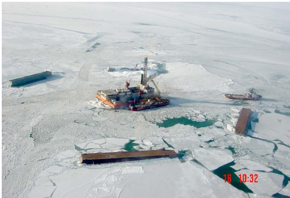
Figure 8-4: Ice management for shallow water drilling / production platform Sunkar by means of ice protection structures and ice breaking vessels (Caspian Sea)
