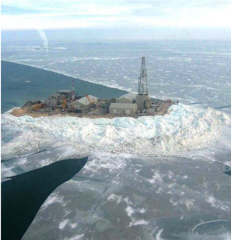
Figure 8-3: Massive ice built-up at a shallow water production platform under influence of ice drift (Caspian Sea)
