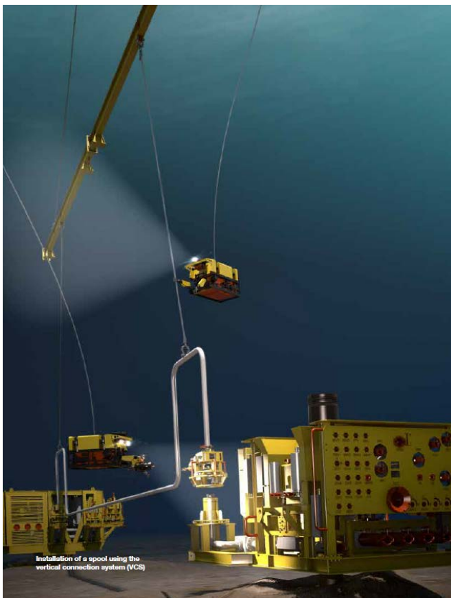
Figure 11-17: Vertical installation of subsea spool pieces (artist impression, Aker Solutions)
