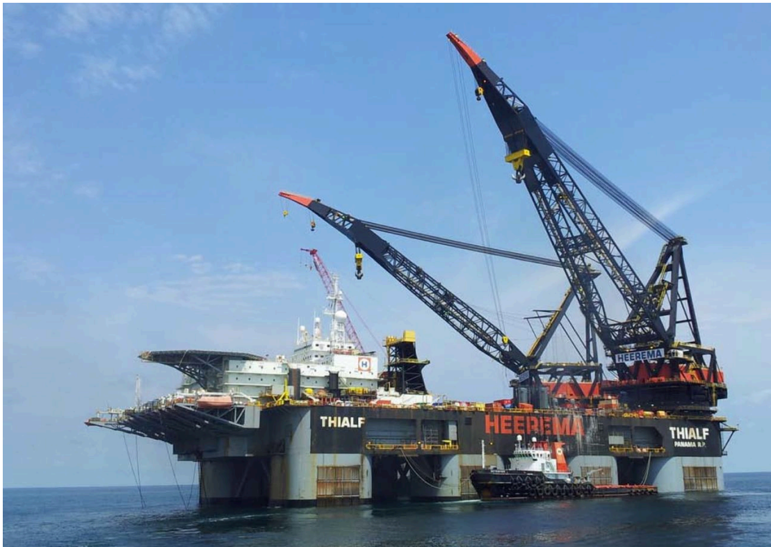
Figure 11-12: Super heavy-load construction vessel (semi-submersible 'Thialf') with crane capacity up to 14.000 t (2x 7.000 t, Heerema)
